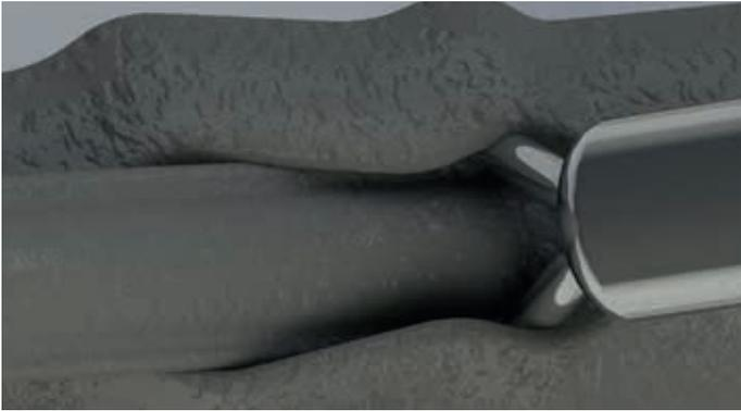
It is now time to fit the filler strip. Before doing this pour a small amount of diluted washing up liquid in the channel that it is to be fitted. Starting at the middle of the bottom, insert the glazing tool into the groove and place the filler strip into the loop of the tool. Run the tool around the groove following the length of filler strip. This should now be placing the filler strip into the groove.
