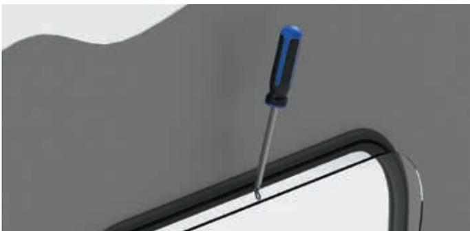
The next step is to remove your window. This can be done by inserting the glazing tool into the top middle face of the seal and pushing around the back of the window. The window can then be levered forward towards you and lifted away. The old seal can now be removed.
